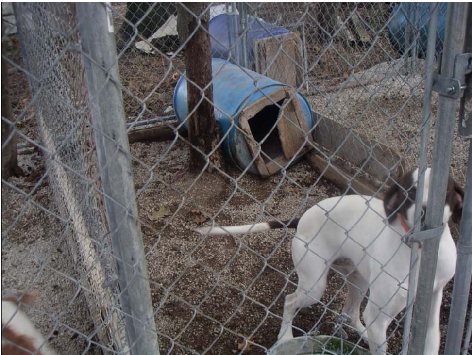
Barrel Shelter: Inadequate Space; No Wind/Rain Break; Untreated, Broken, and Chewed Wood
